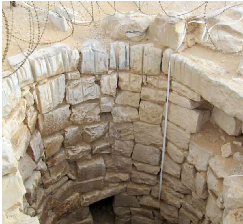
The well at Rehoboth
